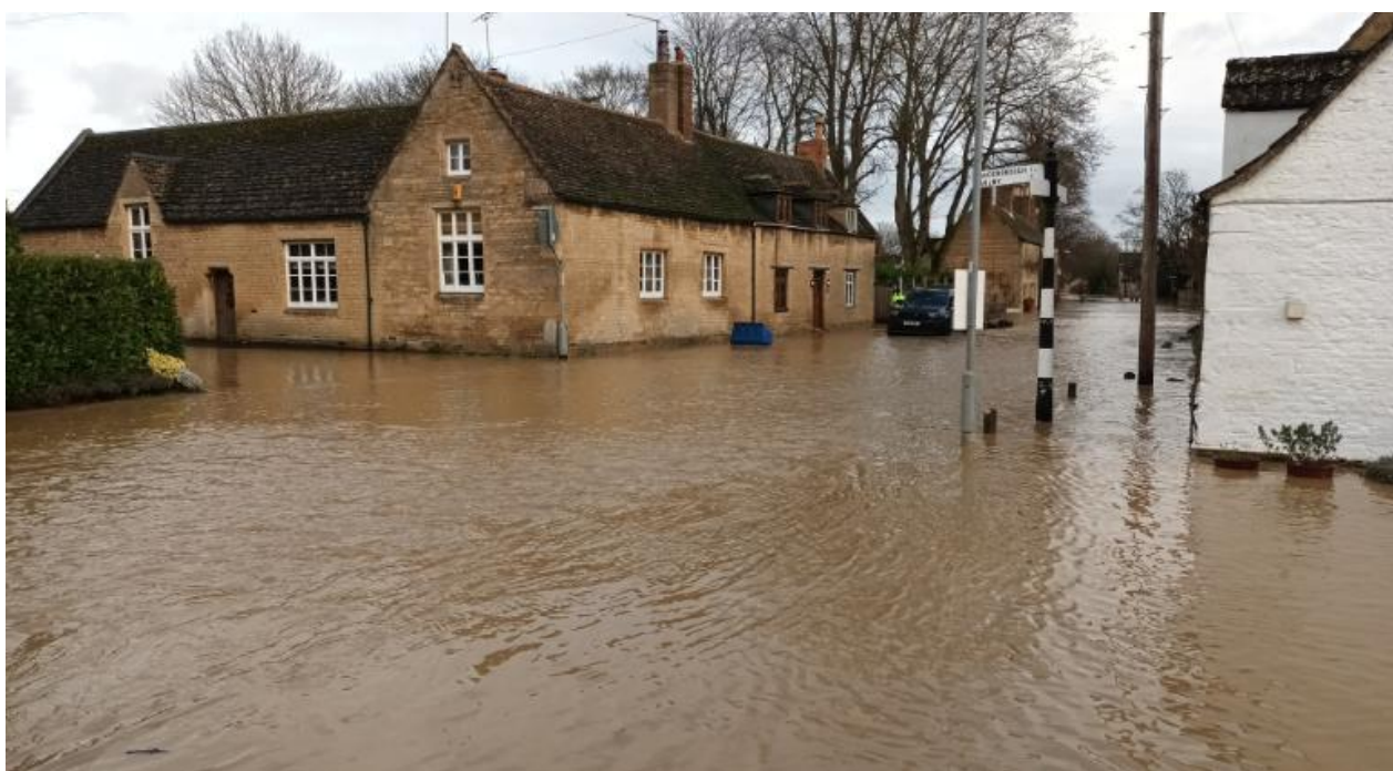
The T junction at Greatford Main St facing the Old School House
