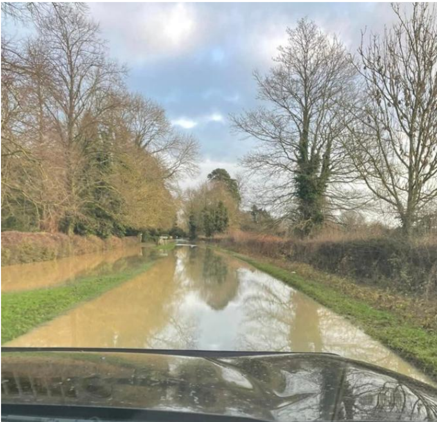
The road into Greatford from the Shillingthorpe gauge, now a river
